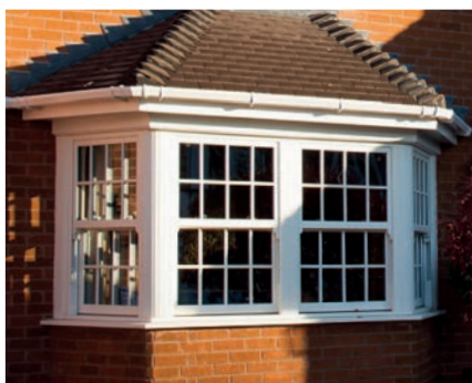
Bay window with vertical sliding sash windows
